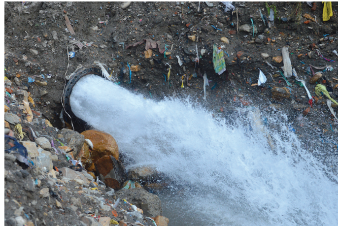
■ Flushing of the Bulk Distribution System in progress on the banks of the Manohara river in Lalitpur (Report on Page 2).
